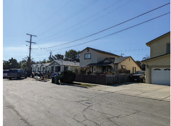
Photo 3: Single-family residence, primary façade and northeast elevation, looking southwest. ICF 2022.
