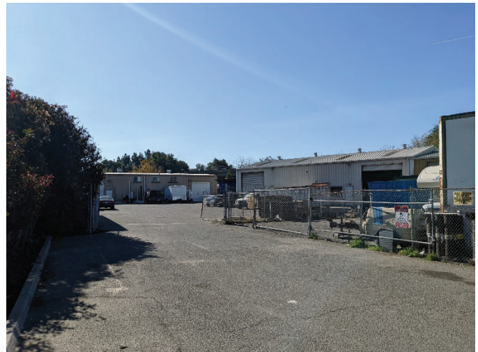
Photo 4: View from Von Euw Common towards the east elevation of building five and the north elevation of building six, looking southwest. ICF. 2022.
