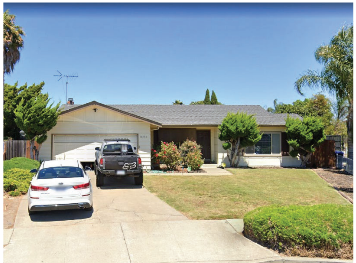
Photo 3 36304 Beech Place, House Type 2, looking N. Google. 2022.
