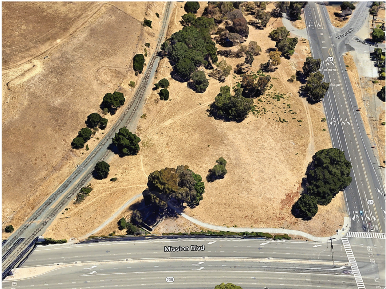
Photo 5. Vallejo Mill Historical Park with stone foundation at center-left, Niles Canyon Railroad Historic District line at left, intersection of Mission Boulevard and Niles Canyon Road/SR 84, looking northeast
