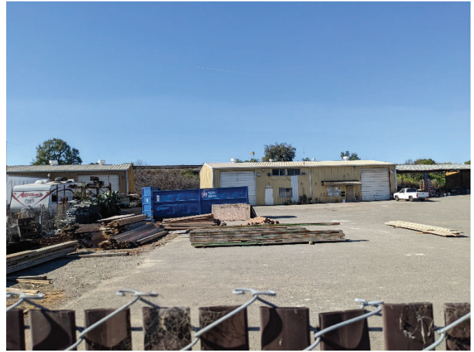
Photo 2: View of the east elevations of buildings three and four, with open storage space and materials in the foreground, looking west. ICF. 2022.
