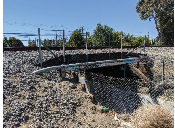
Photo 3: Detail view of east elevation of bridge and abutments. ICF 2022.
