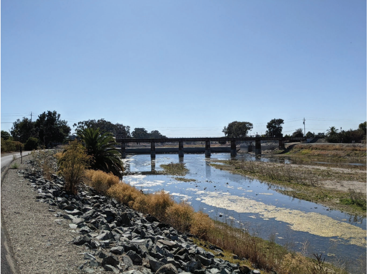
Photo 4. Alameda Creek looking west to the East Union Pacific Alameda Creek Railroad Bridge from the Alameda Creek Trail
