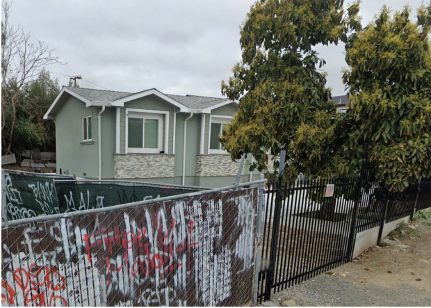
Photo 2: Single-family residence, primary façade and southeast elevation, looking northwest. Google 2021.
