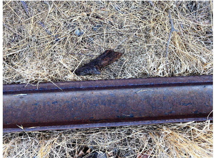
Photo 2: Close up view of 1924 side track (on its side). ICF 2022.
