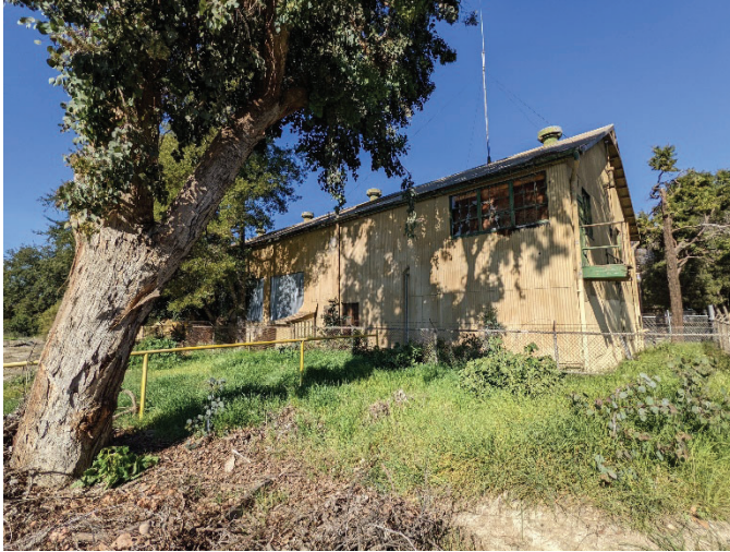
Photo 3: View of the south elevation, looking northwest. ICF 2022.
