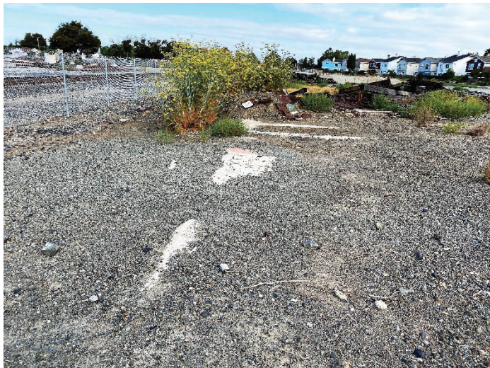
Photo 9 View northwest, concrete pad from demolished depot at southwest corner of parcel. Active UPRR tracks at left. ICF 2022.
