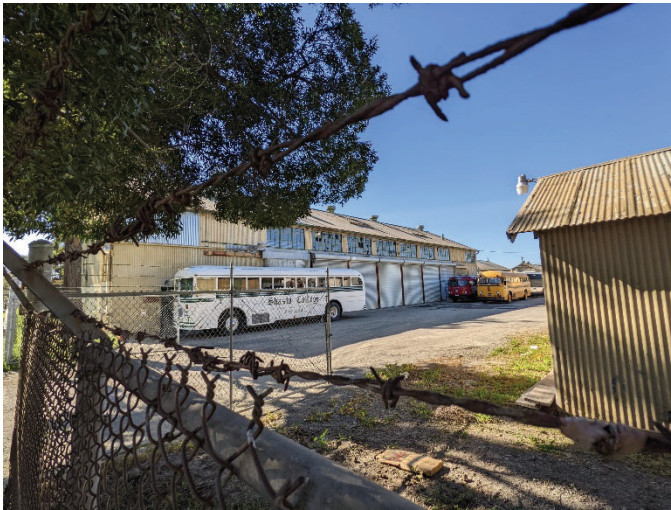
Photo 1: View of the north elevation, looking southwest. ICF 2022.
