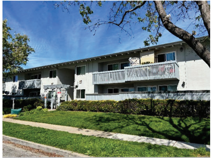
Photo 3 West elevation of an apartment building with small pergola from Bettencourt Street, looking NE. ICF. 2023.
