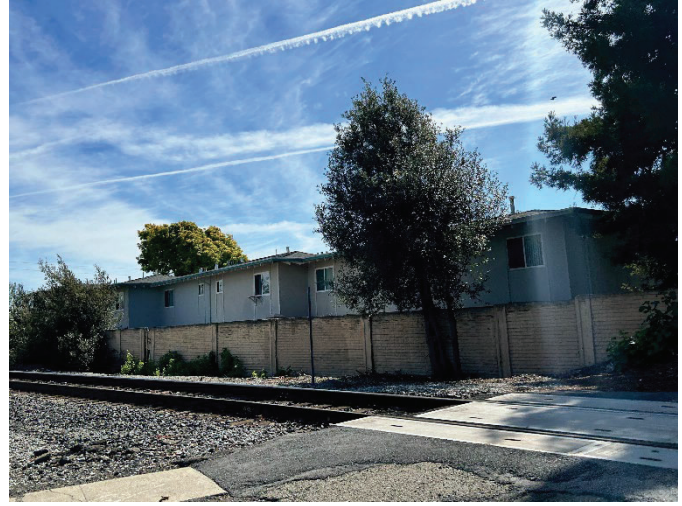
Photo 6 East elevations and eastern property boundary, lined by a concrete block wall across Haley Street and the railroad tracks, looking SW. ICF. 2023.
