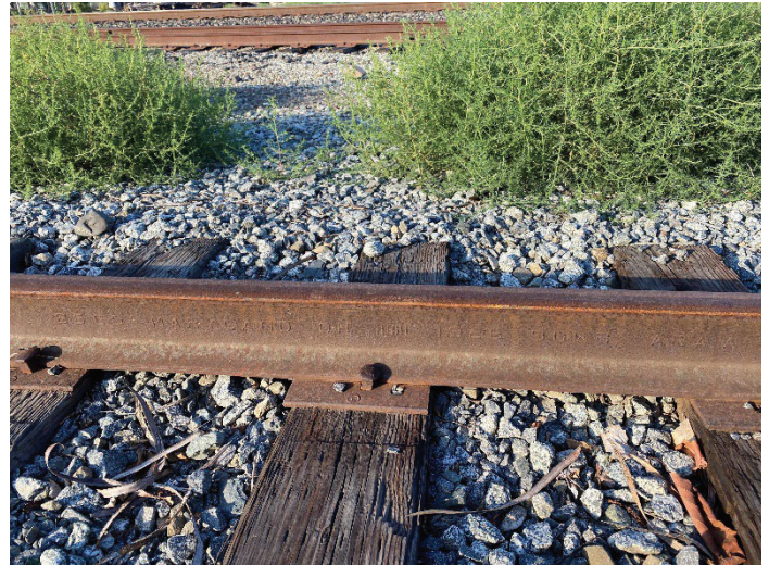
Photo 6: Close up view of 1926 side track. ICF 2022.
