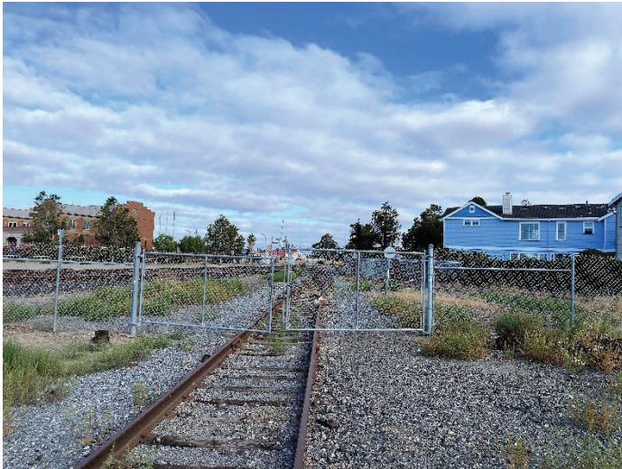
Photo 5: View northwest showing side track dating to 1926 with modern fencing. ICF 2022.
