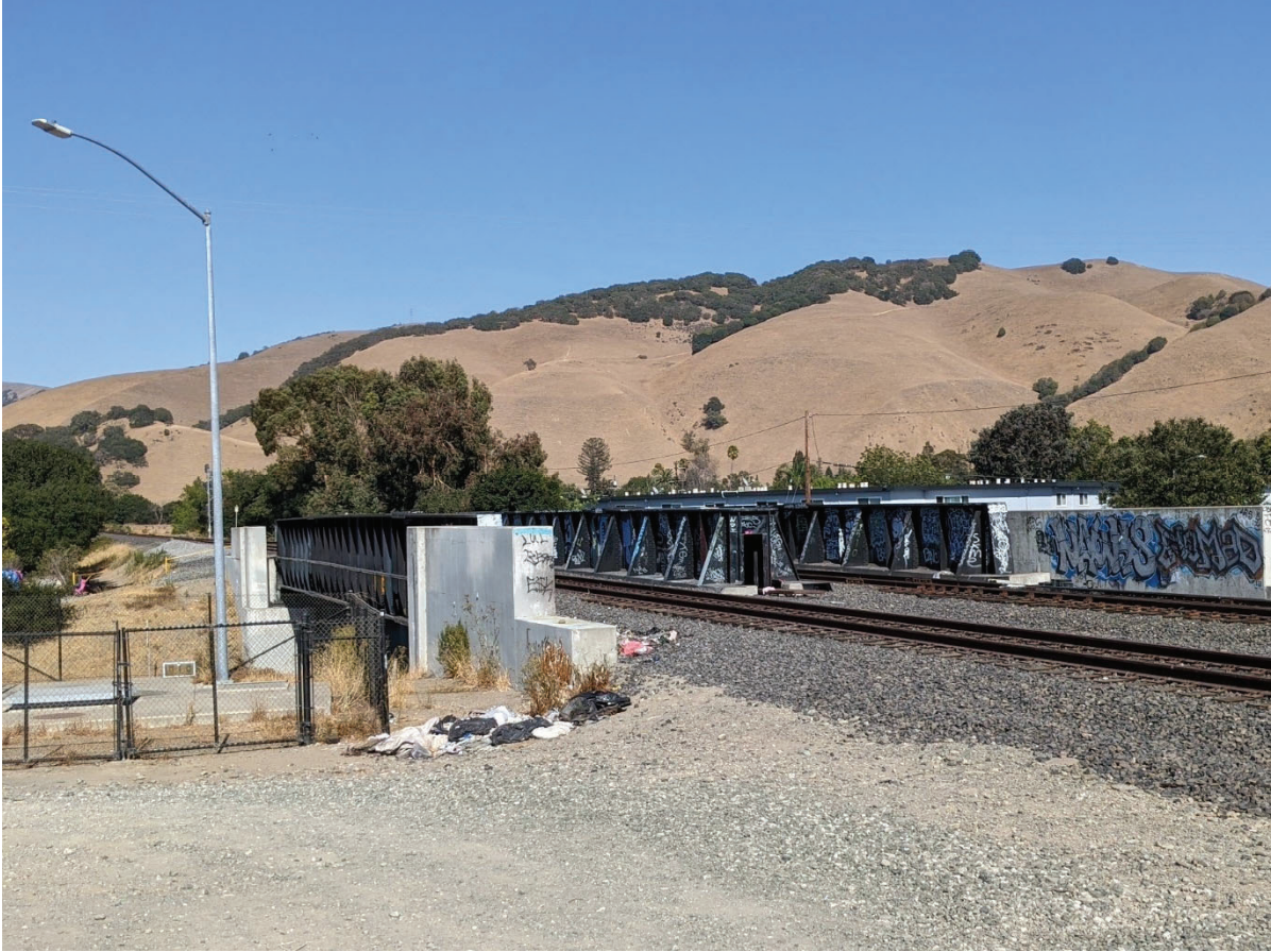
Photo 8. Western Pacific Railroad at Mission Boulevard, looking east
