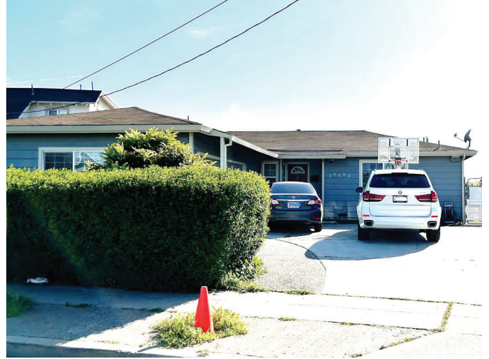
Photo 7 36363 Colbert Street, House Type 2, view south. ICF. 2023.
