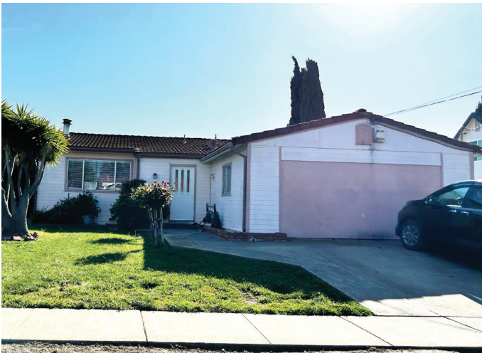
Photo 8 36493 Colbert Street, House Type 3, view south. ICF. 2023.
