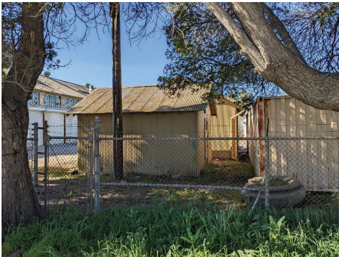
Photo 5: Additional buildings adjacent to the primary Pacific Bus Museum building, looking southwest. ICF 2022.
