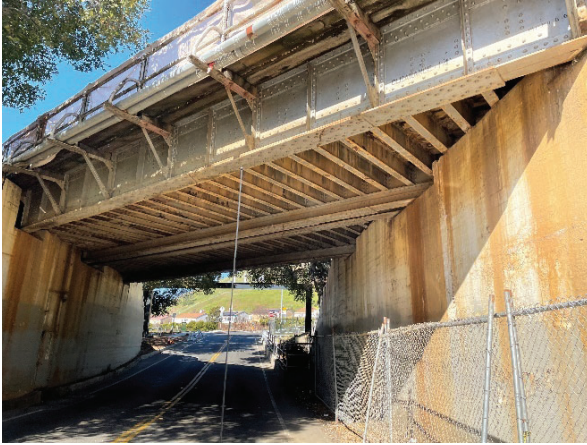
Photo 2: Detail view of underside of deck. ICF 2022.
