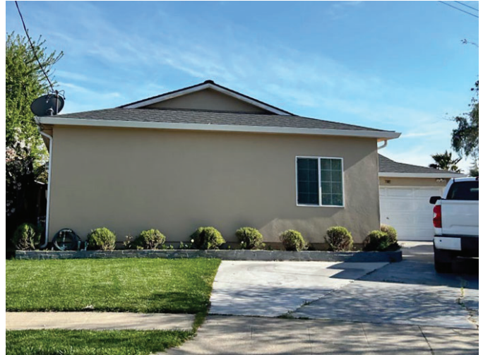
Photo 3 7198 Calais Place, House Type 1, looking SE. ICF. 2023.
