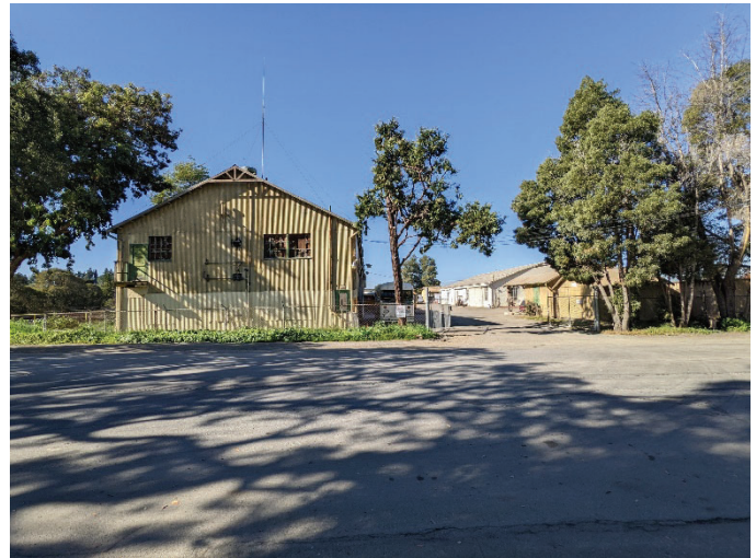
Photo 2: View of the east elevation, looking west. ICF 2022.
