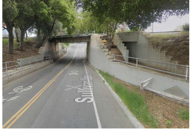
Photo 3: North elevation of the bridge. Google 2021.
