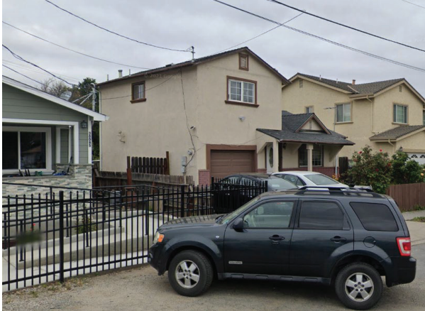
Photo 2: Single-family residence, primary façade and southeast elevation, looking northwest. Google 2021.
