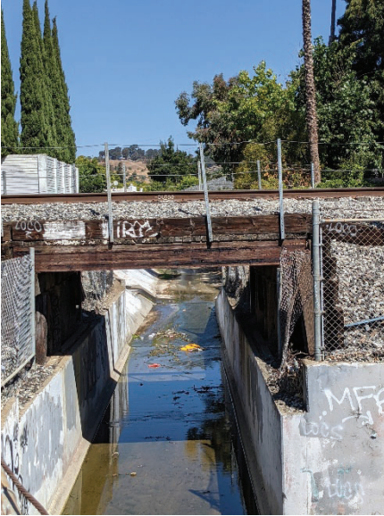
Photo 2: East elevation of the bridge. ICF 2022.
