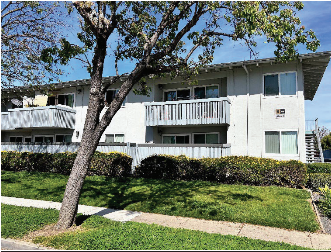
Photo 2 West elevation of an apartment building from Bettencourt Street, looking NE. ICF. 2023.
