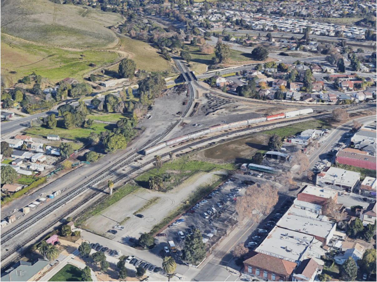
Photo 1. Niles Canyon Railroad Historic District wye, looking east towards Niles Canyon from Niles
