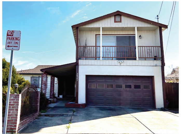
Photo 5 36347 Colbert Place, House Type 4, looking S. ICF. 2023.
