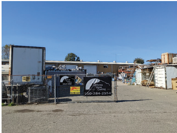
Photo 3: View of the east elevation of building four, partially obstructed by open storage space and materials in the foreground, looking west. ICF. 2022.
