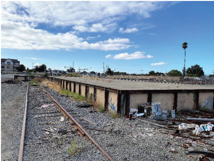
Photo 7 View southeast showing concrete foundation and 1926 side tracks. ICF 2022.
